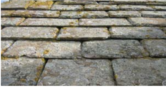
Traditional weathered slate roof
