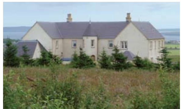
New-build Laird House
