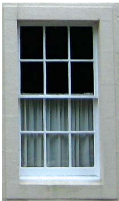
Traditional six-over-six pane window
