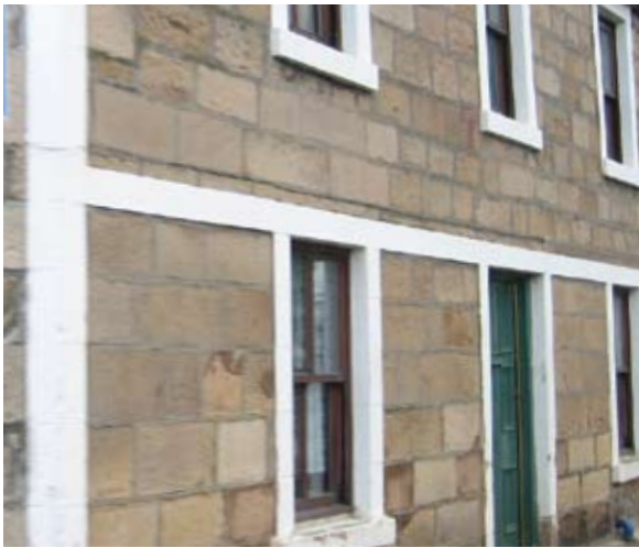
Typical granite wall with render trim
